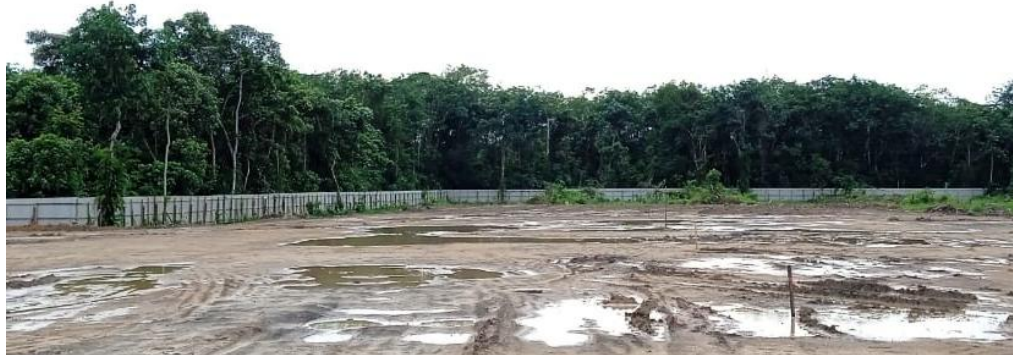
Figure 2. Rain Halts Work
