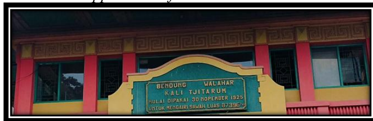
Ornamental Tessellation on the Upper Wall of the Walahar Dam
