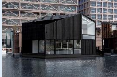
Figure 2. Building view from the river
