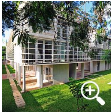
Figure 11. Building view from courtyard
