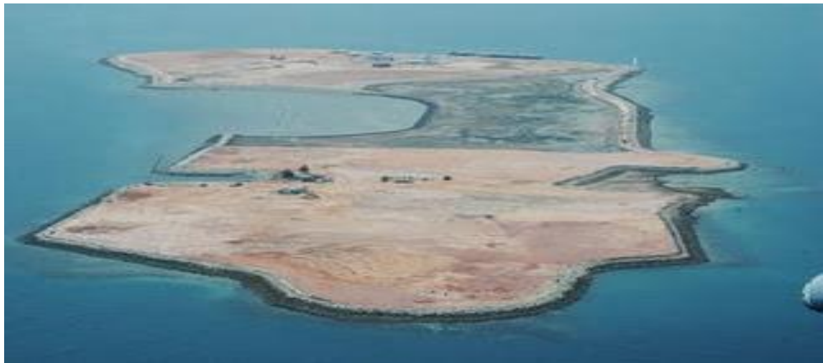
Image 4. Nipa Island after Reclamation
