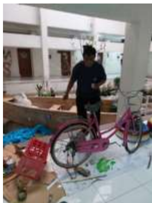
Gambar 5. Persiapan material outdoor communal space
